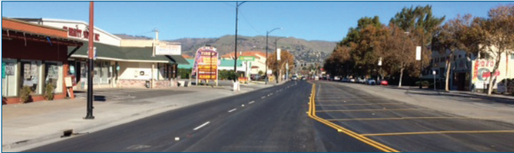
Newly paved lanes on westbound Alum Rock Avenue
